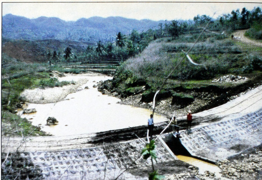
Using available building materials, Rus helps a community in the dry area of Central Java build a dam to conserve the little rainwater they get during the wet season.
