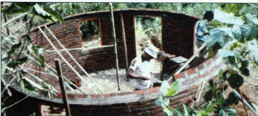
In a remote area of Irian Jaya, Rus introduces circular brick-wall construction to the Dani tribe. The solid walls of the new structures offer much better protection against the weather than the tribe's traditional huts.
